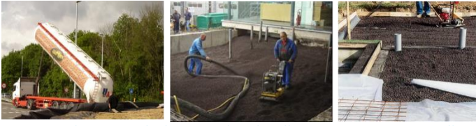
Figure 3: Blowing and vibrating plate levelling compactation installation
