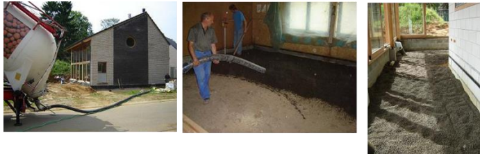
Figure 4: Blowing with manual levelling installation
